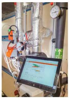
Evaluation of the recorded data to optimise delta T and the V<sub>max</sub> value in the roof ventilation centre.
